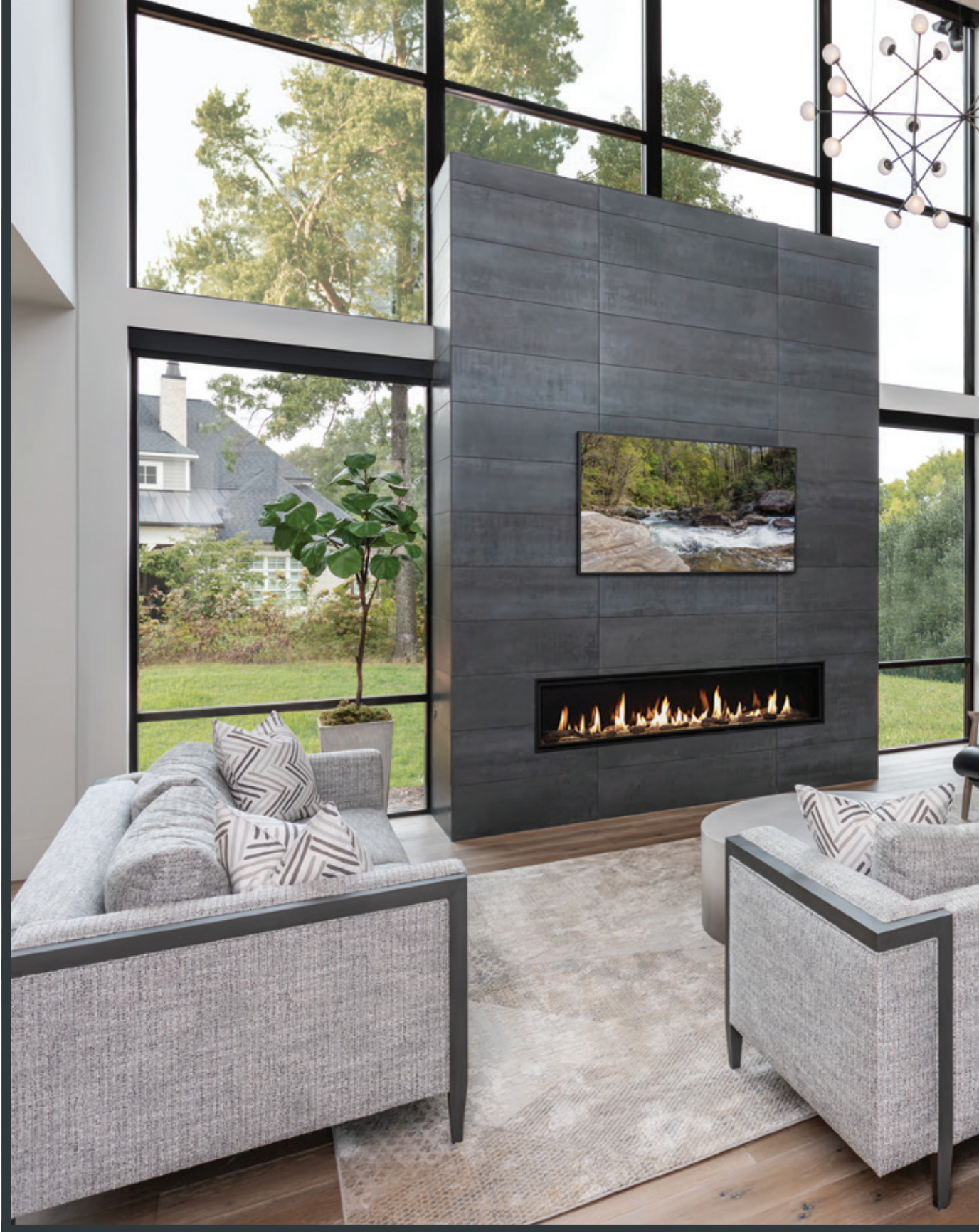
The custom fireplace is direct vent gas with an exterior brick wall and an interior composed of long-format linear tiles. A frame television embedded over the flames can display art or any form of network entertainment.
